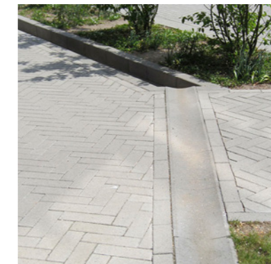
Concrete water channel
