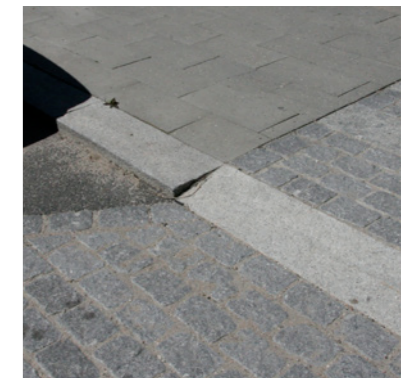
Granite curbstone around planting
