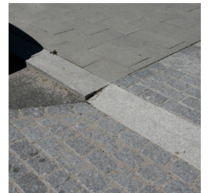
Granite curbstone around planting
