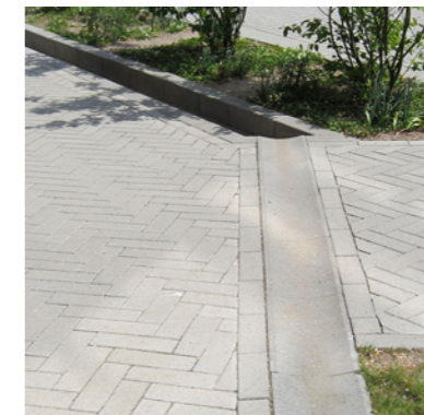
Concrete water channel
