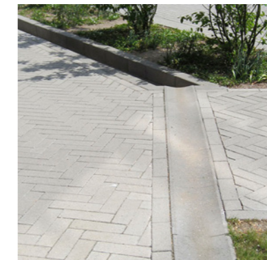
Concrete water channel
